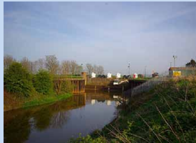
Drainage System in Hull: Bransholme Pumping Station
