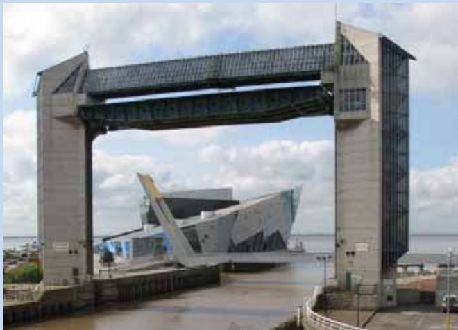
Flood Defences in Hull: The River Hull Tidal Barrier
